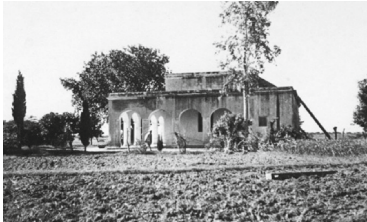
Kothi house near the Beas railway station
